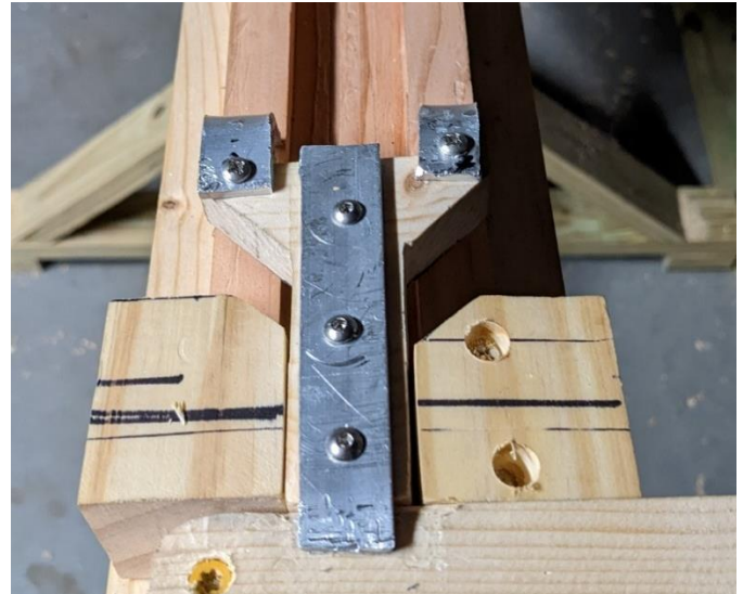
Figure 25: Top View of Repair
